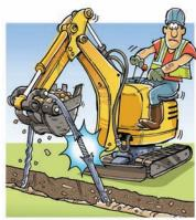
It is also important to note that underground cables can be found anywhere and not just in highways and footpaths, so major excavations should not start until you have checked with us that there are no cables in the vicinity of your work.
