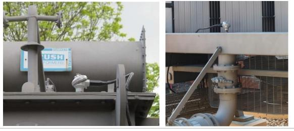
Figure 5 : Illustration of top of tank and bottom of cooler oil temperature sensor
