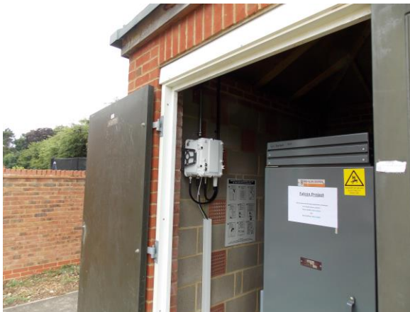
Figure 11: Typical Ground Based Secondary Site Installation
