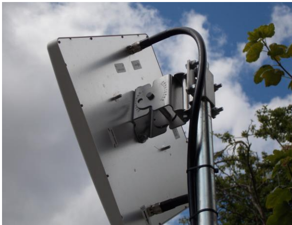
Figure 27: Typical FALCON Panel Antenna (1.4GHz WiMAX)
