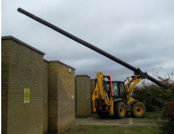
Figure 23: 15m Wood Pole Installation Work
