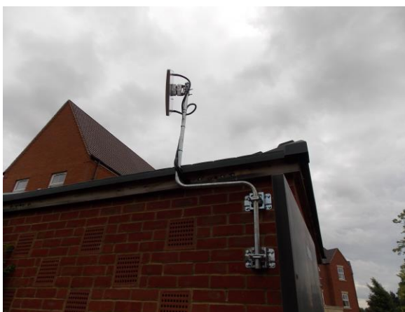
Figure 13: FALCON Antenna on Cranked Pole
