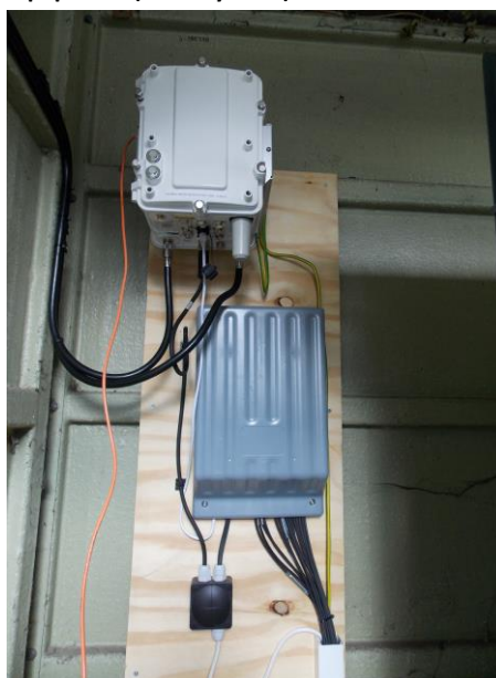
Figure 14: Cisco CGR1240 Router with Attached Equipment (Gridkey LVM)
