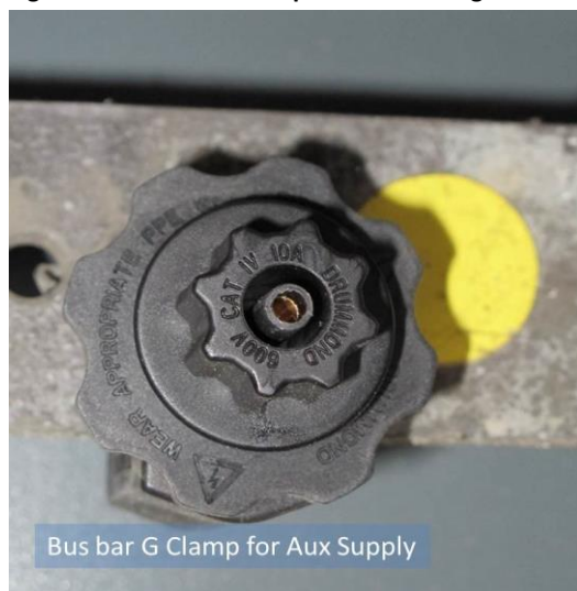
Figure 25: LV Busbar Clamp Power Sourcing
