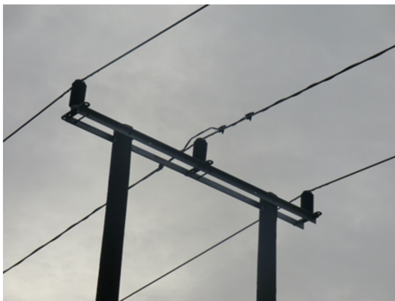
Figure 15 – Rebuilt line with fibre wrap
