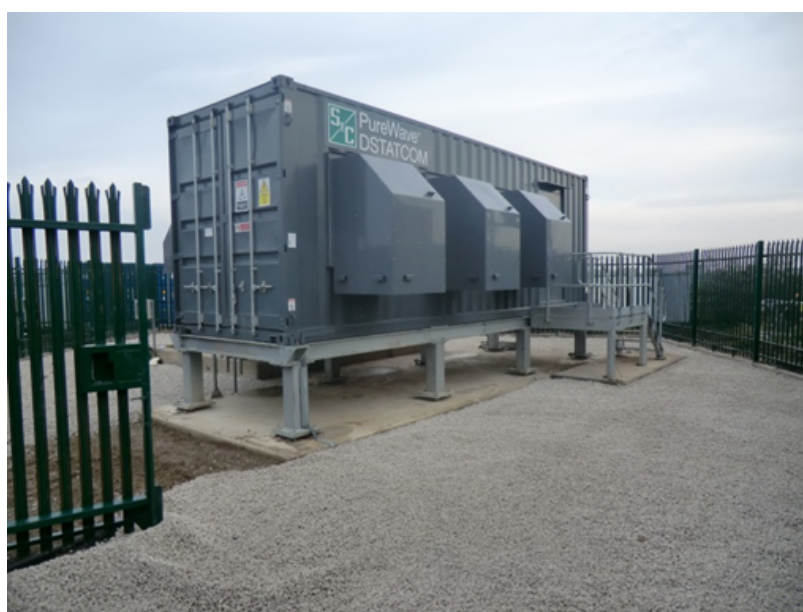
Figure 21 - DStatcom at Trusthorpe primary substation
