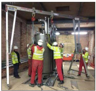
Figure 2-11: Placement of L2 cryostat vessel in its final position on the first floor
