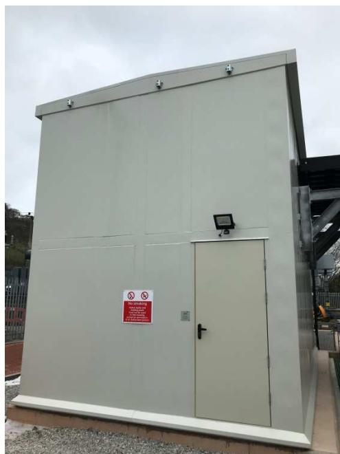
**Figure 2-14: Transformer Noise Enclosure**
