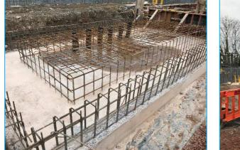
Figure 2-24: Rebar for transformer plinth
