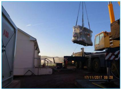
Figure 2-28: Delivery of transformer
