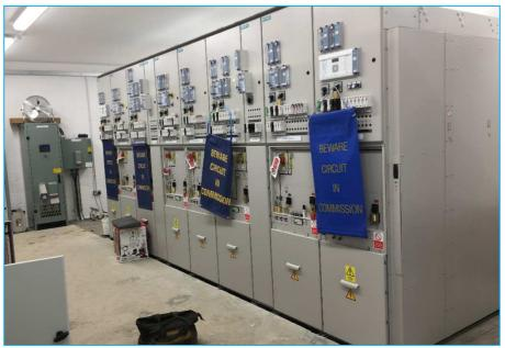
Figure 2-26: 33kV switchboard being commissioned
