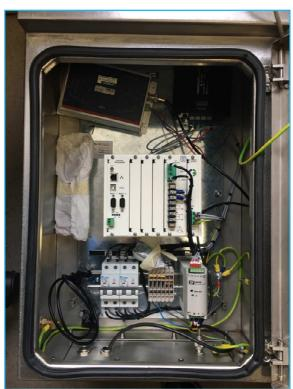
Figure 2-12: Inside of Monitoring panel during testing
