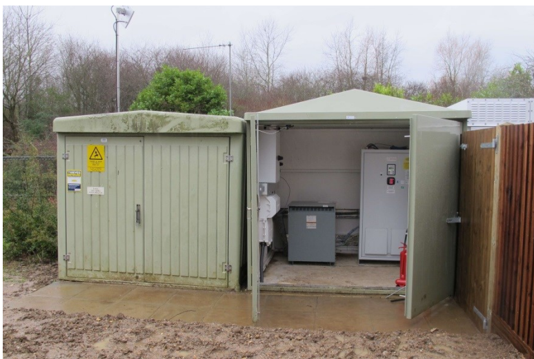
Figure 2.15: 50 kW, 100 kWh EES Installation as part of Project FALCON (Source: WPD)
