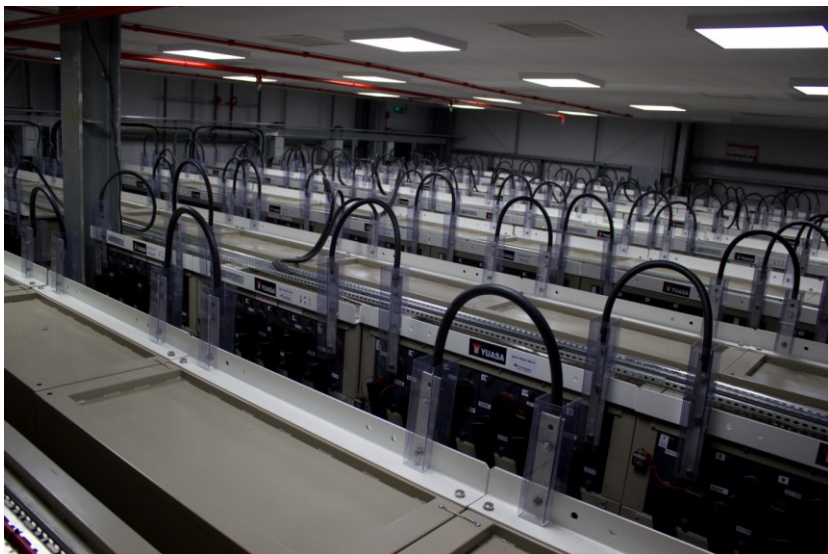
Figure 2.13: 1 MW, 3 MWh EES at Lerwick, Shetland (Source: SSEPD)
