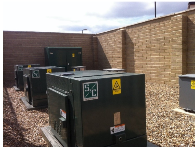
Figure 2.8: 3x 25kW, 25kWh ESS at Chalvey, Slough (Source: SSEPD)
