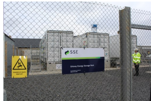
Figure 8.3: 2MW/500kWh EES System (SSEPD) - Containerised
