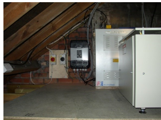
Figure 8.5: 2kW/4kWh Residential EES System (WPD) - Installed within domestic loft spaces
