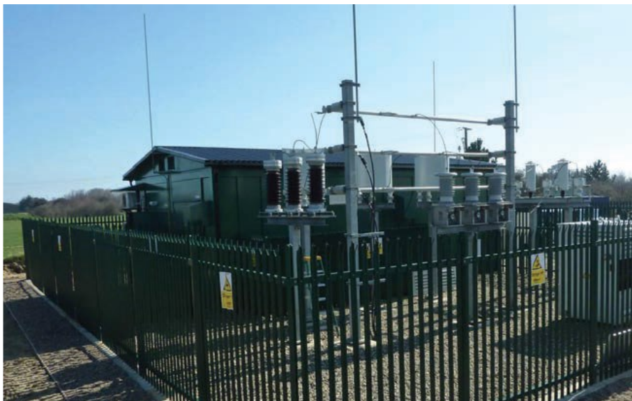
Figure 2.7: 200 kW, 200 kWh ESS at Martham, Norfolk (Source: UK Power Networks)
