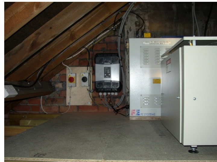
Figure 2.14: 2 kW, 4 kWh Domestic EES Installation as part of SolaBristol (Source: WPD)
