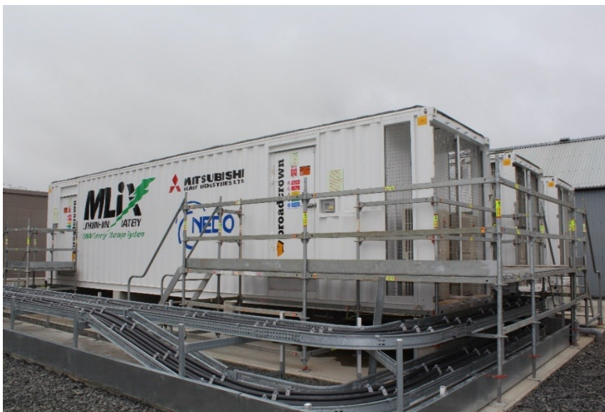
Figure 2.5: 2 MW, 500 kWh ESS at Kirkwall, Orkney (Source: SSEPD)
