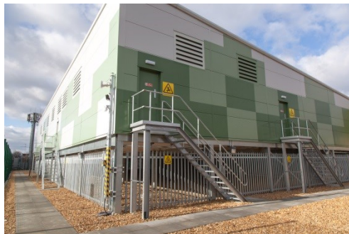
Figure 8.2: 6MW/10MWh EES System (UKPN) - Installed in a purpose built building
