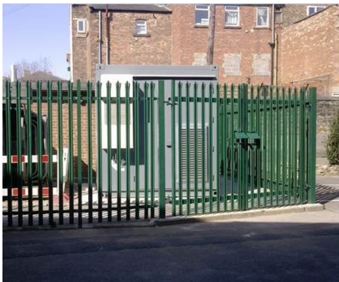
Figure 2.11: 100 kW, 200 kWh ESS at Darlington (Source: Northern Powergrid)
