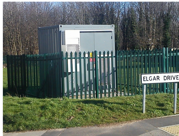
Figure 2.10: 50 kW, 100 kWh ESS in Sheffield (Source: Northern Powergrid)
