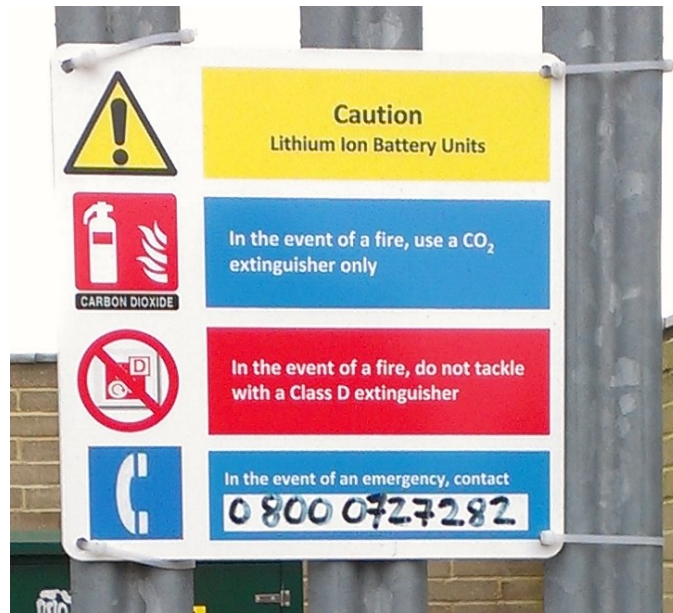
Figure 9.2: Example Fire Fighting Guidance Sign (Photograph by EA Technology)
