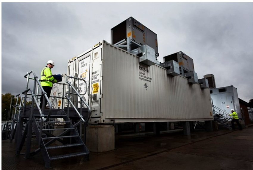
Figure 2.9: 2.5 MW, 5 MWh ESS at Darlington, Co. Durham (Source: Northern Powergrid)
