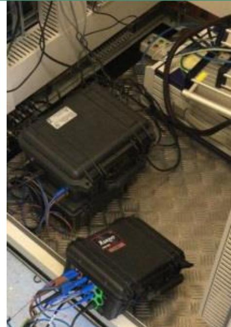
*Above: Example of Power Quality monitoring equipment installed inside a 33kV substation.*
