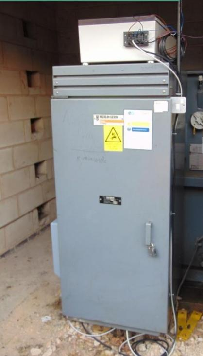
*Above: Recent installation completed in Derby. The white box mounted on the top of the LV cabinet is the OpenLV equipment. Bottom left of the cabinet is the grey LucyGridKey monitoring box.*
