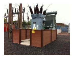
Since 2010 we have been designing for flood risk at all our new substations, including smaller distribution substations. The usual mitigation for a new site is to place equipment on raised plinths to ensure it remains above the predicted level of any flooding.
