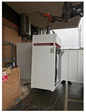
Figure 11: Battery Units Lifted by Crane
