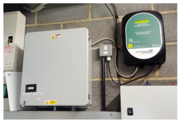
Figure 18: Controller Installation at WPD Boston Depot; Tesla Powerpack Site Master Controller is on the left, Nortech Controller is on the right.
