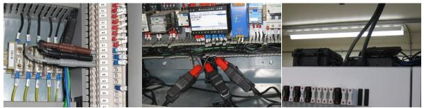
Figure 2-1 – Pilot PQ monitor installation at Meaford C. From left to right: connections in to VT secondary wiring; current clamps around CT secondary wiring; Envoy communications hub and PM7000 PQ monitor installed on top of switchgear.
