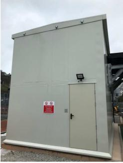
Figure 2-14: Transformer Noise Enclosure
