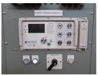
Figure 50-2: GT2 SuperTAPP relay and Controls
