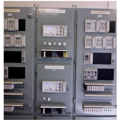
Figure 42-1: Replacement Front Doors Containing SuperTAPP SG Relays
