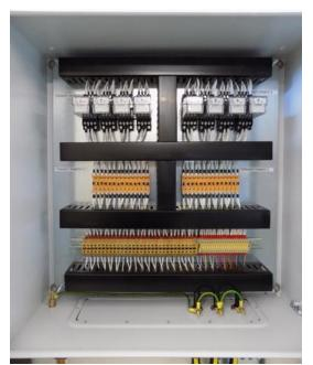
Figure 2-19: MicroTAPP SVO Control Panel Wiring at Waterlake Primary Substation
