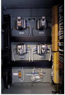
Figure 42-3: Internal Auxiliary Relays for T1
