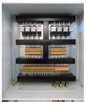
Figure 70-2: SVO Control Panel Internals
