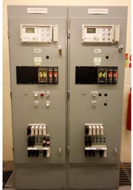
Figure 46-1: T1 and T2 Modified Tap Change Panels
