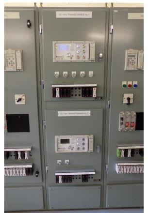
Figure 38-1: Replacement Front Doors containing SuperTAPP SG
