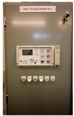
Figure 10-3: Detail of GT1 SuperTAPP SG Installation
