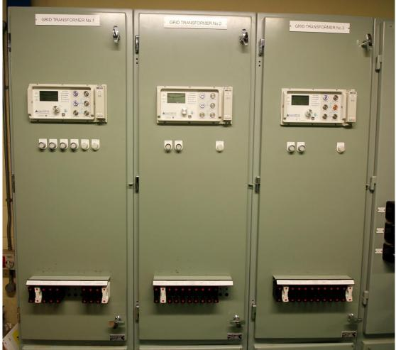
Figure 58-1: GT1, GT2 and GT3 Tap Change Panels with SuperTAPP SG Relays Installed
