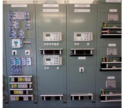
Figure 14-1: GT1, GT2 and GT3 SuperTAPP SG Installation
