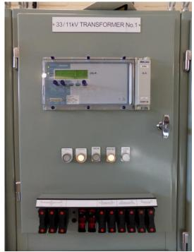
Figure 70-1: SVO Control Modifications to T1 Panel
