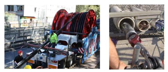
Figure 4.13: Pulling of HTS cable into the ducts [16]
