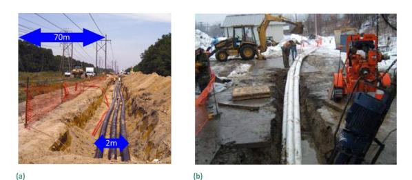
Figure 4.9: (a) Long Island 138 kV 575 MW HTS cable flat laying configuration (b) Three-in-one cable laying configuration [21]
