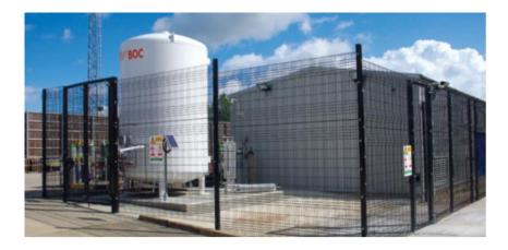
Figure 4.17: Outdoor secure liquid nitrogen storage [35]
