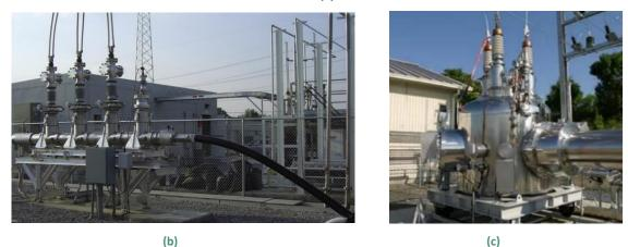
Figure 4.5: Superconducting cable terminal configuration (a) three single-phase termination, (b) three-in-one termination, and (c) triaxial termination
