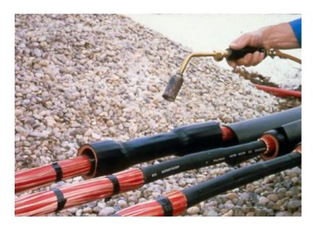
Figure 5.3: Raychem heat shrink cable joint
