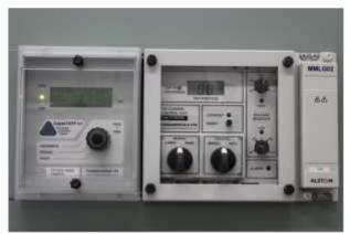
Figure 2-6: Fundamentals SuperTAPP N+ AVC Relay
