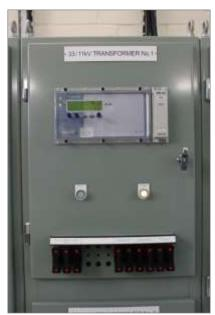
Figure 2-8: MicroTAPP AVC Relay
