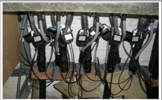
Figure 51: Sub-station feeder Sensors
