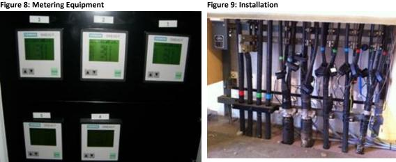
Figure 8: Metering Equipment
