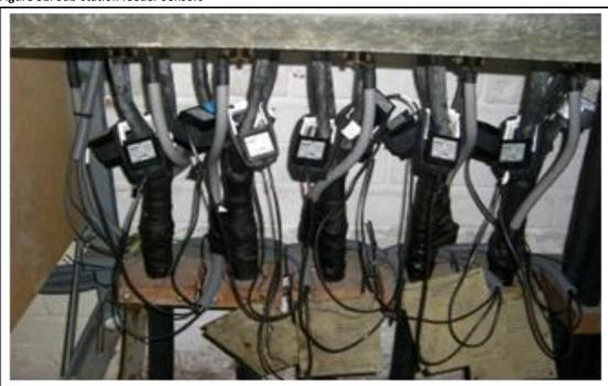
Figure 51: Sub-station feeder Sensors
