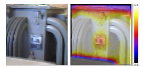
Figure 7: Sample thermal image of an in-service Distribution transformer.
