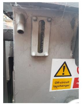
Fig. 1.1 : A typical pole-mounted transformer showing the head-space vent
