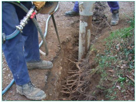
Figure 2-6 Illustration of vacuum excavation method
