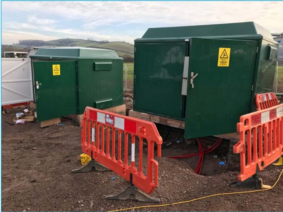
Figure 3-24: LV Substations during Installation
