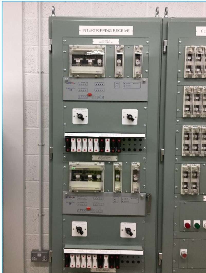
Figure 3-27: Picture of Intertrip Panel at Exebridge
