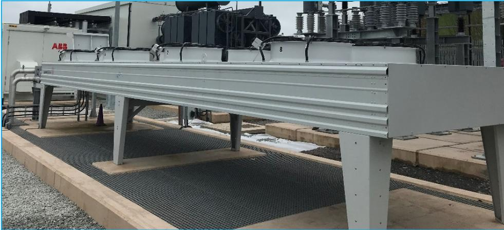
Figure 5-9: Picture of Installed FPL Heat Exchanger
