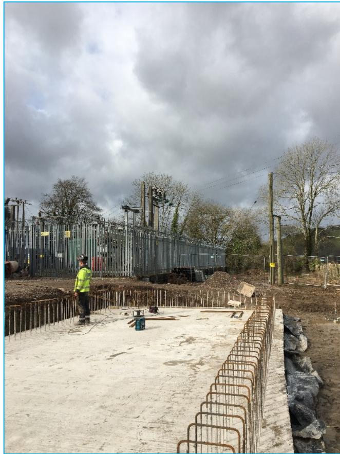
Figure 3-11: 33kV Switchroom Foundation construction
