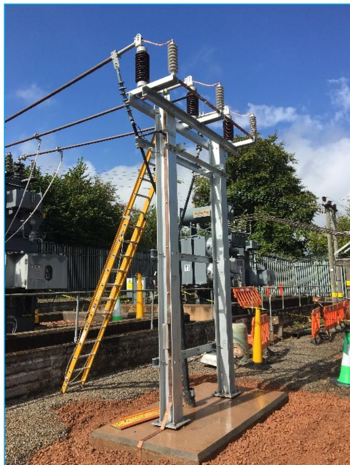
Figure 3-15: Picture of New Transformer HV Termination
