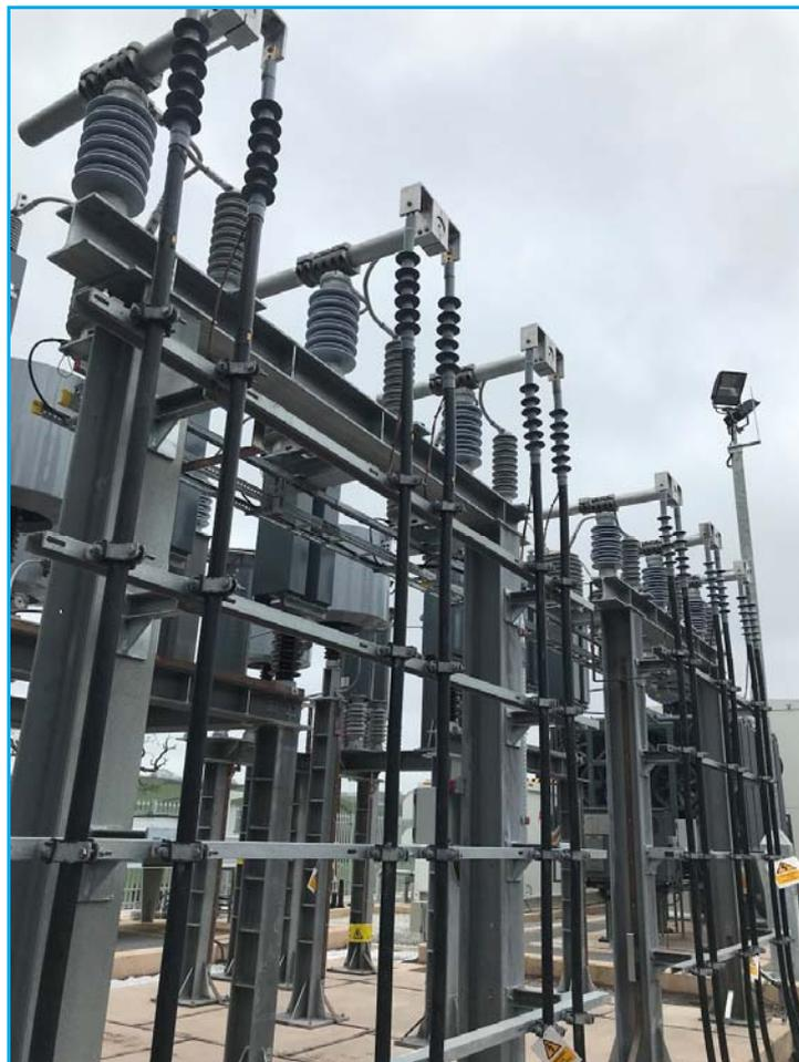
**Figure 5-8: 33kV Terminations to Harmonic Filters**
