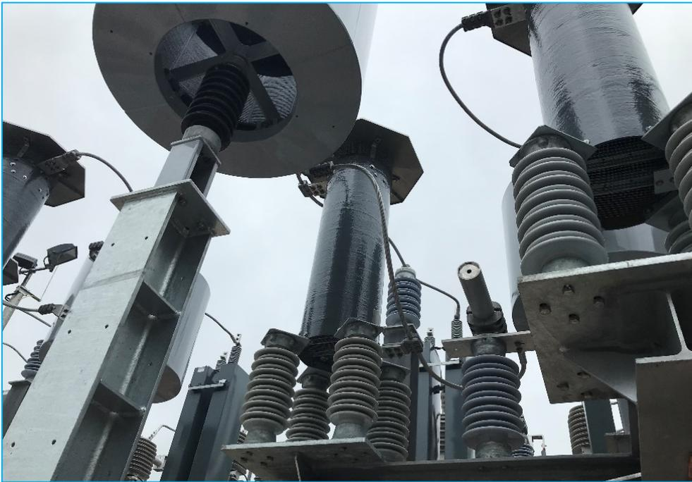
**Figure 5-7: Installed Harmonic Filters**
