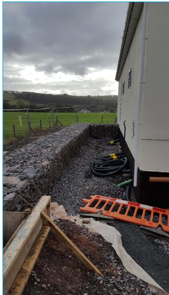
Figure 3-20: New Retaining wall during construction behind new 33kV Switchgear Building
