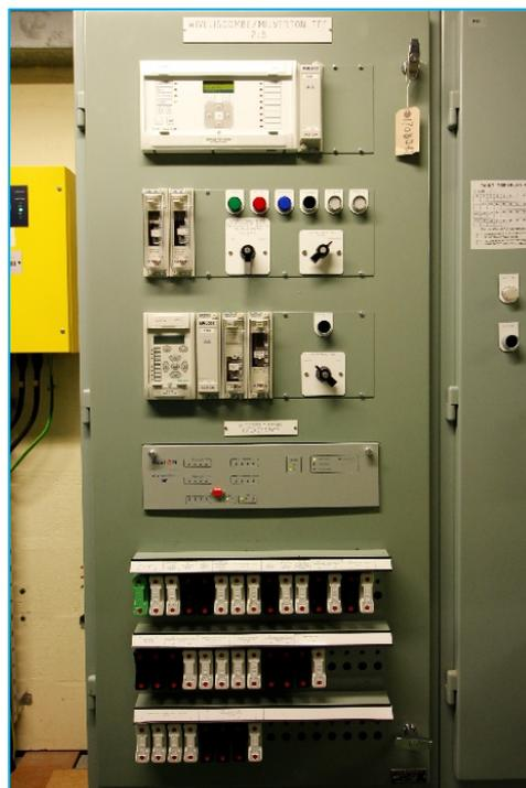
Figure 3-26: Combined Protection and Intertrip Panel at Taunton BSP
