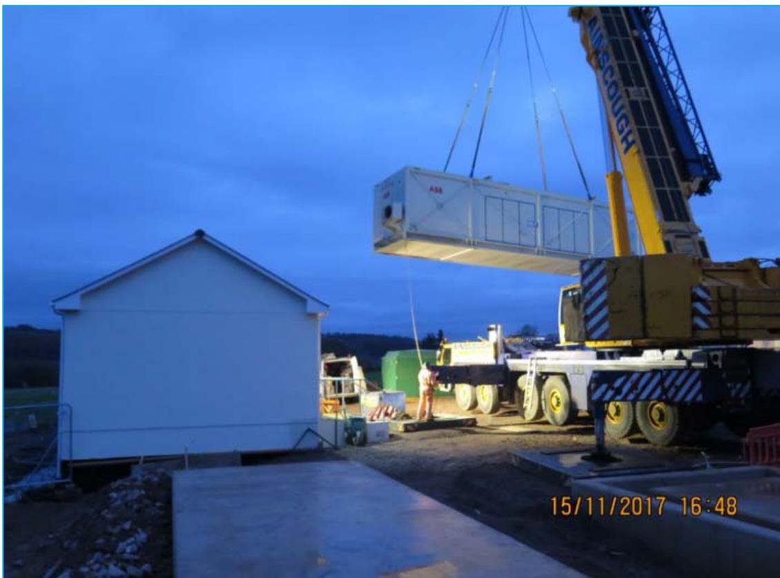
Figure 5-1: Delivery of FPL Converter Container
