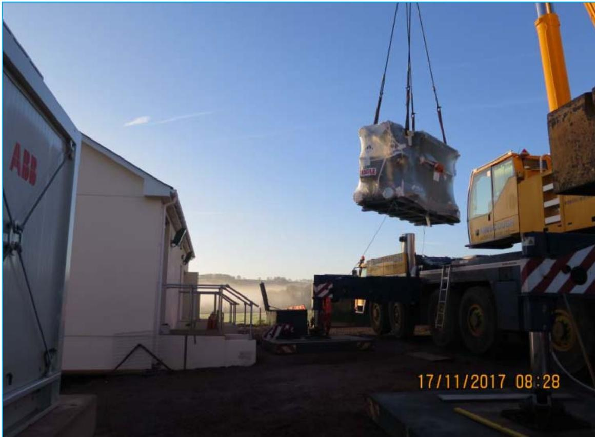
Figure 5-4: FPL Transformer Delivery
