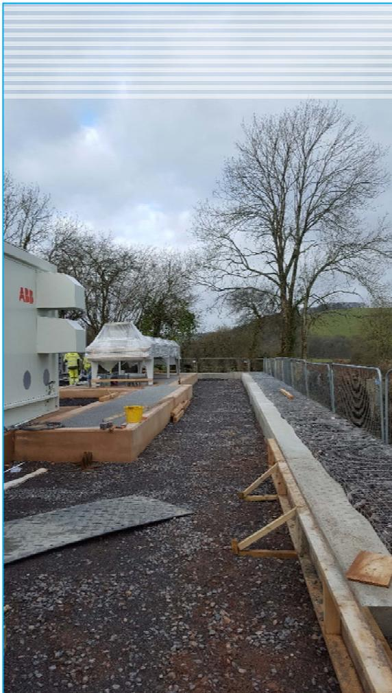
Figure 3-19: New Retaining wall along 33kV Compound
