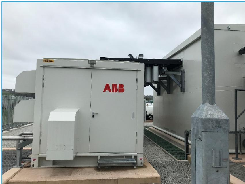
Figure 5-3 Picture of FPL Converter Container and connection to FPL Transformer
