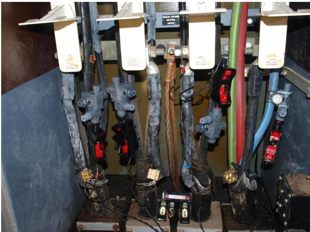
Figure 36: Wavecon cable terminating at fuse board
