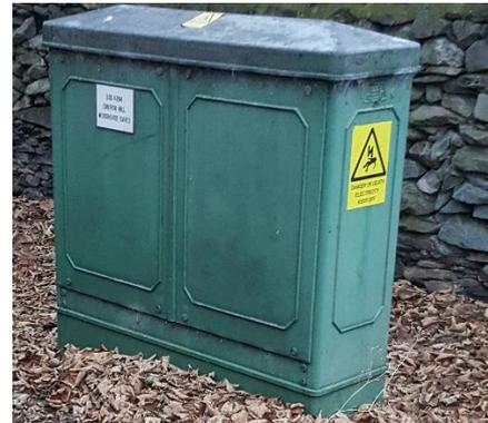
Figure 24 Photograph of LV fuse board (rear view)
