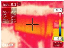
Figure 19 Thermal image of ring main unit
