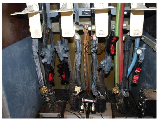
Figure 36: Wavecon cable terminating at fuse board
