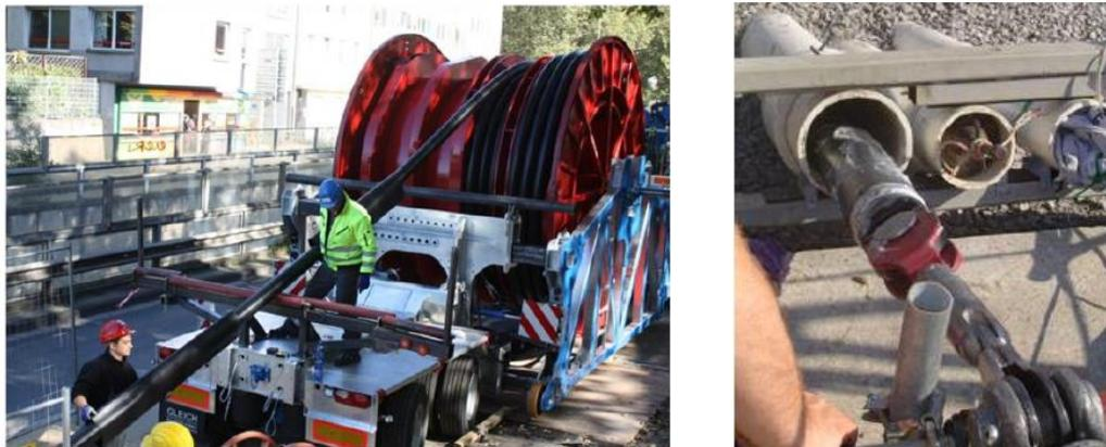
Figure 4.13: Pulling of HTS cable into the ducts [16]
