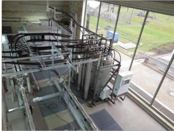
Figure 4.18: Nexans AmpaCity project indoor liquid nitrogen storage
