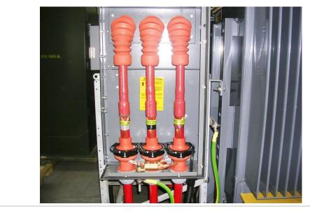
Figure 4 : Installed switchgear CT's.
