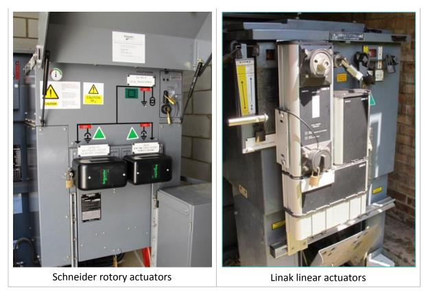
Figure 3 : Installed switchgear actuators.
