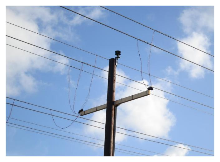
Figure 4 Conductor thermocouple installation
