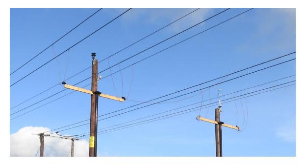
Figure 6 Weather monitoring equipment installed on freestanding intermediate wood poles
