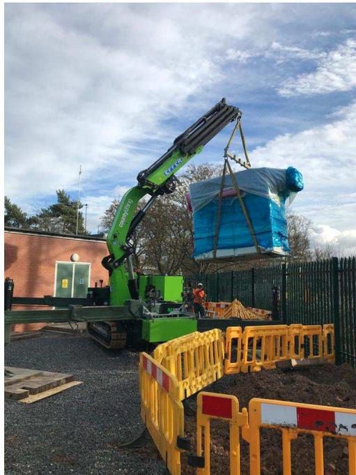
Figure 2-1 Crane offloading FCLi being onto the concrete foundation at UoW
