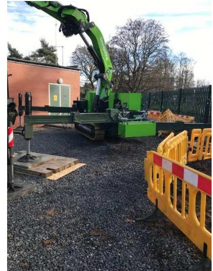
Figure 5-4 Spider crane used for FCLi lift
