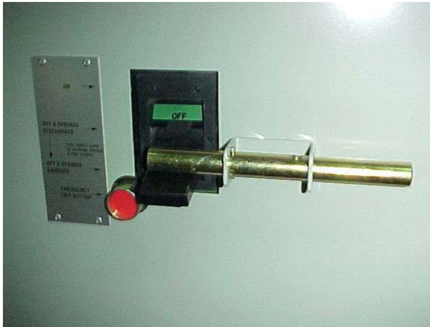
Figure B2 Metering MCCB Locking Arrangement
