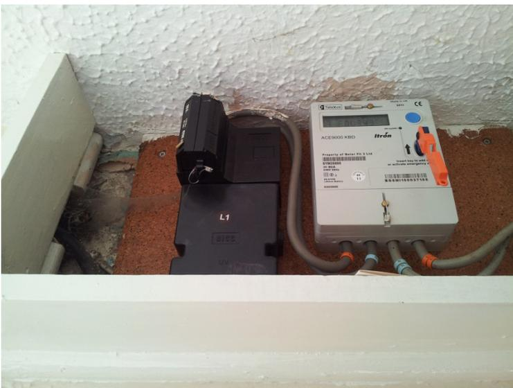
*Figure 61, installation aborted (restricted space photographic evidence)*
