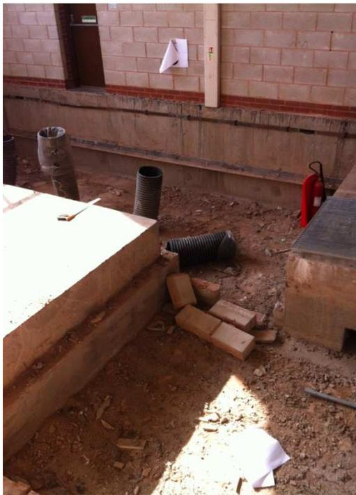
Figure 2-6: Concrete plinth being prepared for extension to accommodate FCL
