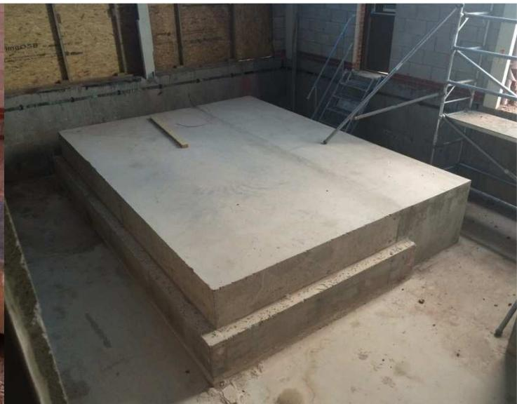
Figure 2-7 - Extended plinth for FCL installation
