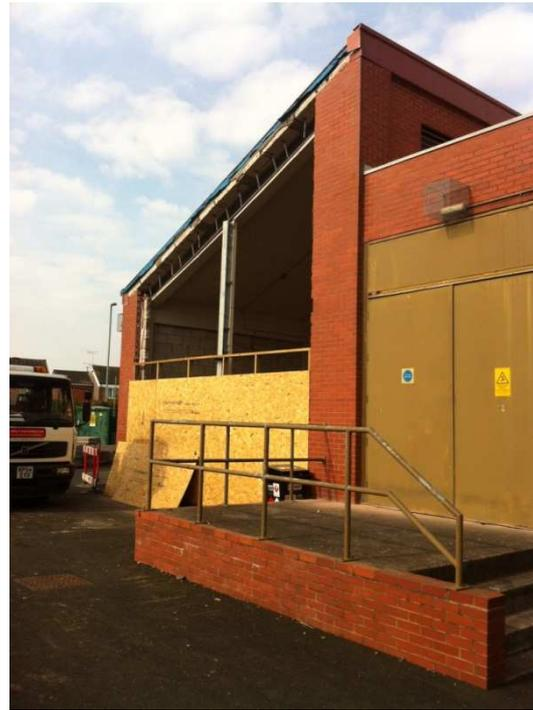
Figure 2-5: Removal of wall ready for FCL installation
