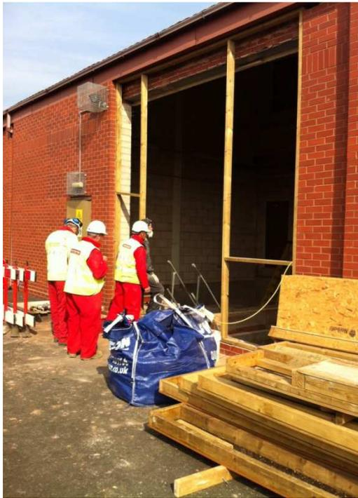
Figure 2-4 - Removal of FLM wall to install equipment
