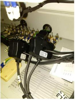
Current sensors on monitored 11kV feeder.
