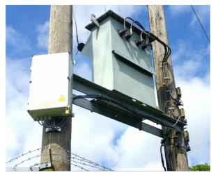
Lucy GridKey MCU 520 monitor at a pole mounted transformer
