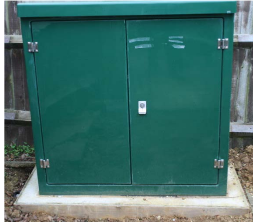
Images 3 & 4.: Meter boxes and GRP housings used for installing ground mounted monitoring
