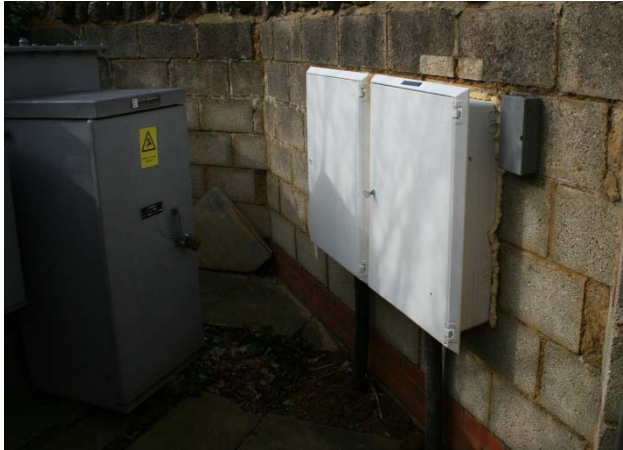
Images 3 & 4.: Meter boxes and GRP housings used for installing ground mounted monitoring
