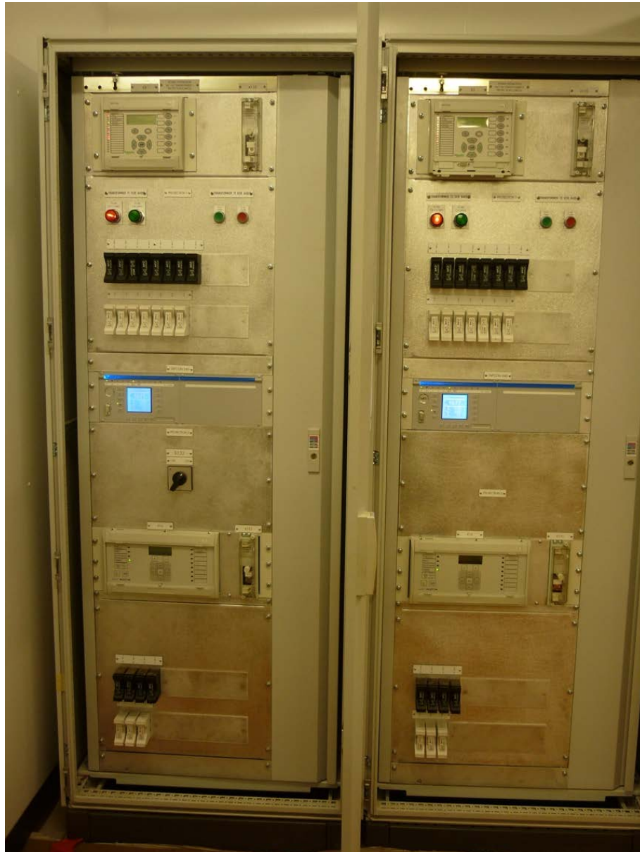
Figure 5-6: TAPCON Typical Panel Mounting
